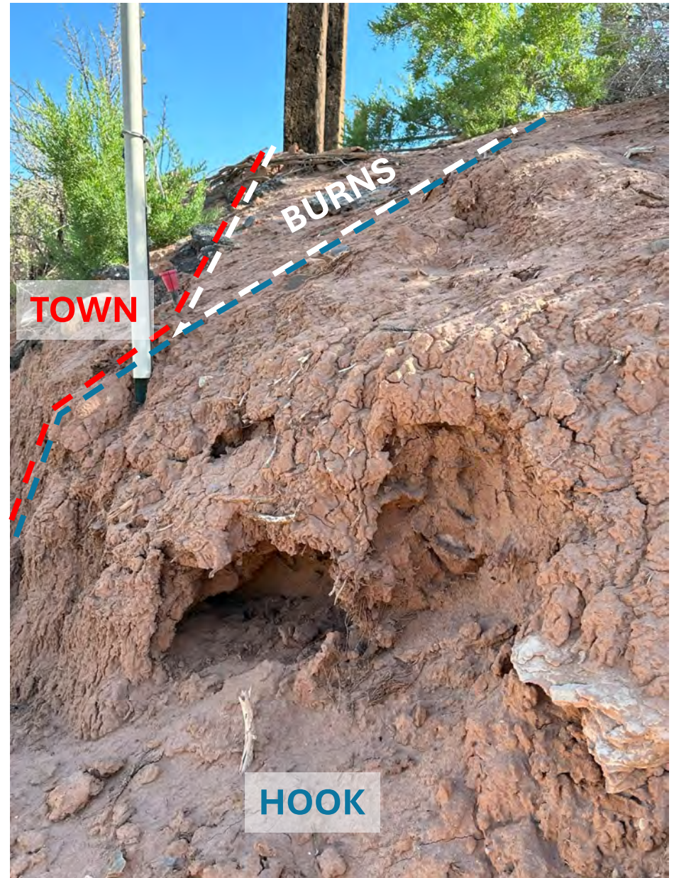
Better view of openings near base of excavated cut where moisture from pipes is exiting and depositing sediment onto trail. Eventually these openings and soil above them will collapse back to swallow holes
